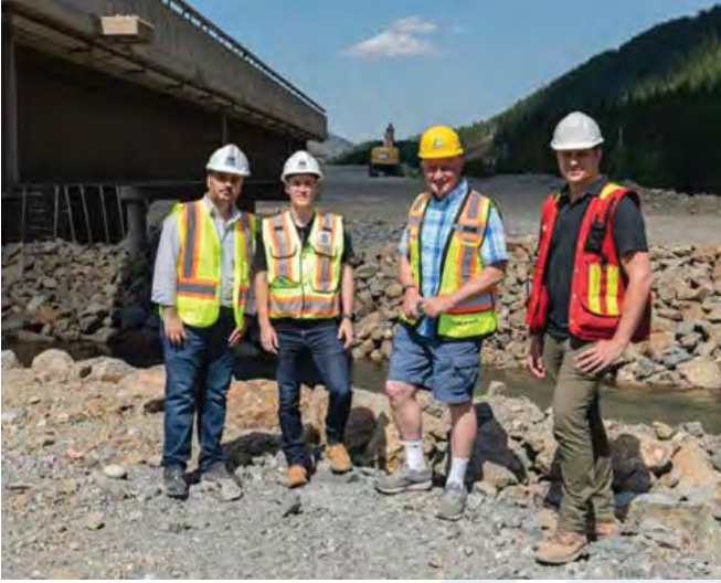
ABOVE: GLP engineers (left to right) Vikram Verma, Dan Cossette and Kent Hodgson with the provincial Minister of Public Safety, the Honourable Mike Farnworth (third from left), in the summer of 2022, inspecting reconstruction of the Coquihalla Highway from damage caused during the atmospheric river the previous year. Credit: Kelly Funk
